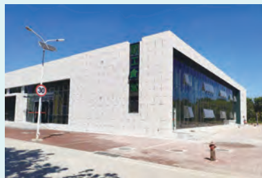
► The newly-built canteen of the Alex Company
